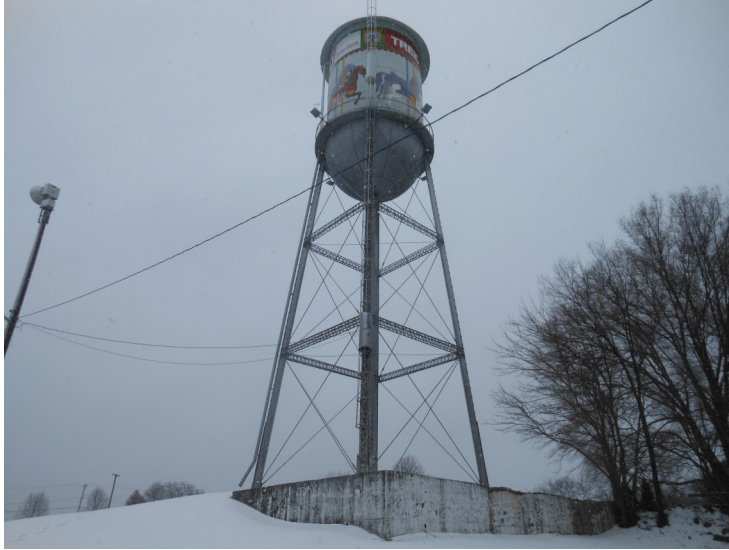
1) 100,000 gallon cone roof elevated water tank located in Waterloo, Wisconsin.
