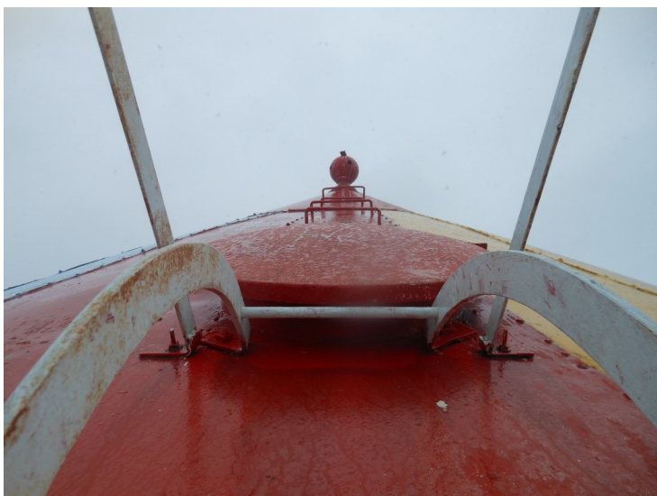
27) There are rungs on the roof leading up to the finial ball at the peak.
