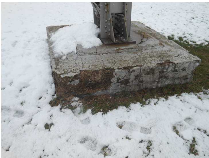
6) Typical concrete leg foundation is in poor condition overall.
