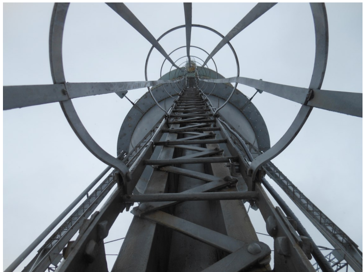
14) The leg ladder is in good condition. The ladder is not equipped with a fall prevention device.
