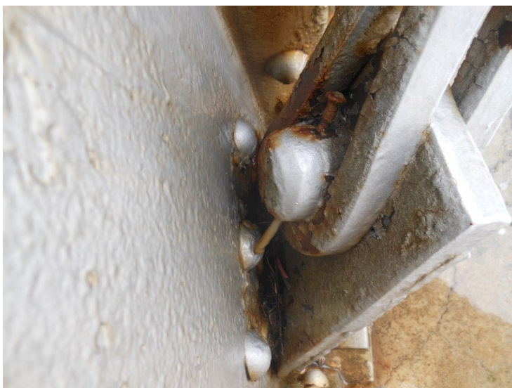
12) Typical sway rod connection is in good condition.
