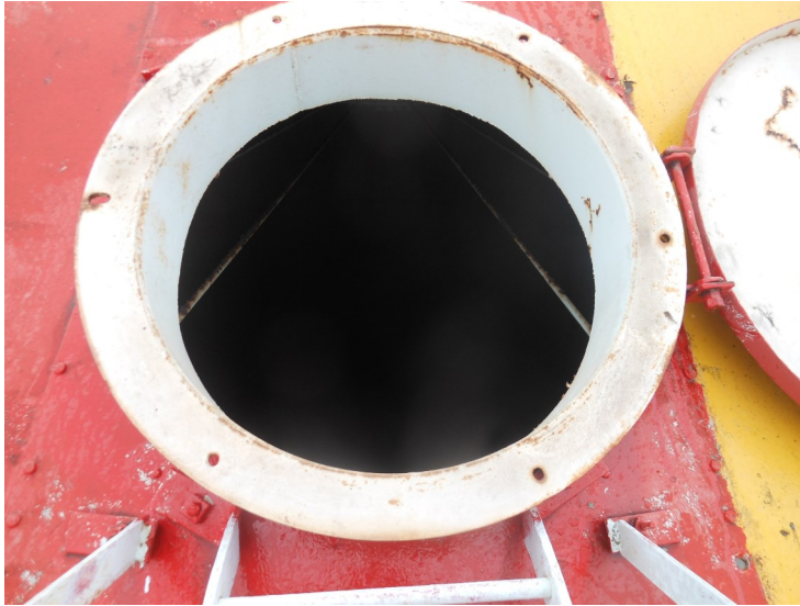
28) The wet interior roof hatch is in good condition.
