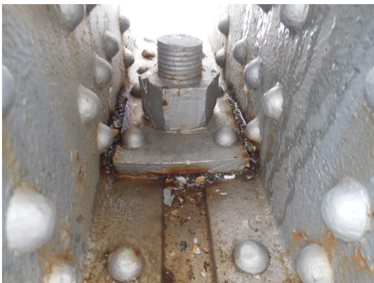
9) Typical leg anchor bolt is in good condition.
