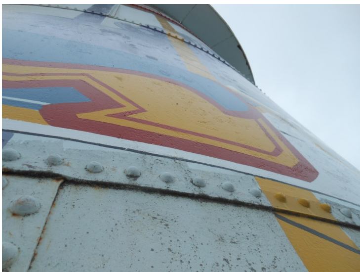
24) The riveted seams on the sidewall are in good condition.
