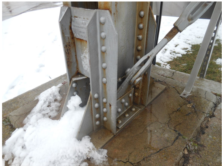
11) Typical leg base is in good condition.
