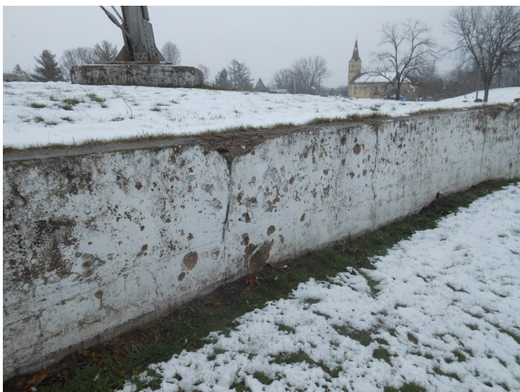
3) The concrete retaining wall is in fair condition with numerous spalls.
