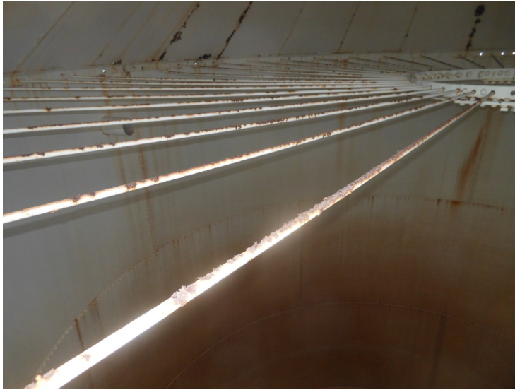
31) The wet interior spider rods are in good condition.
