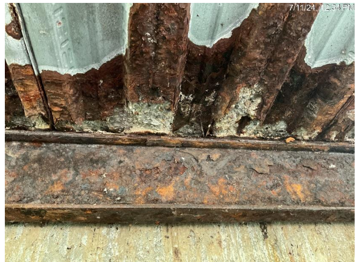
Concrete spall/exposed reinforcing steel at North SIP forms
