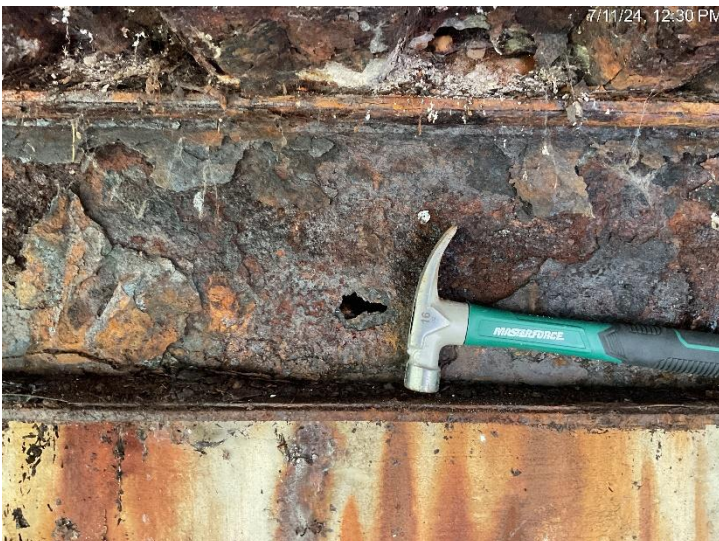
Section loss and corrosion at North floor beam
