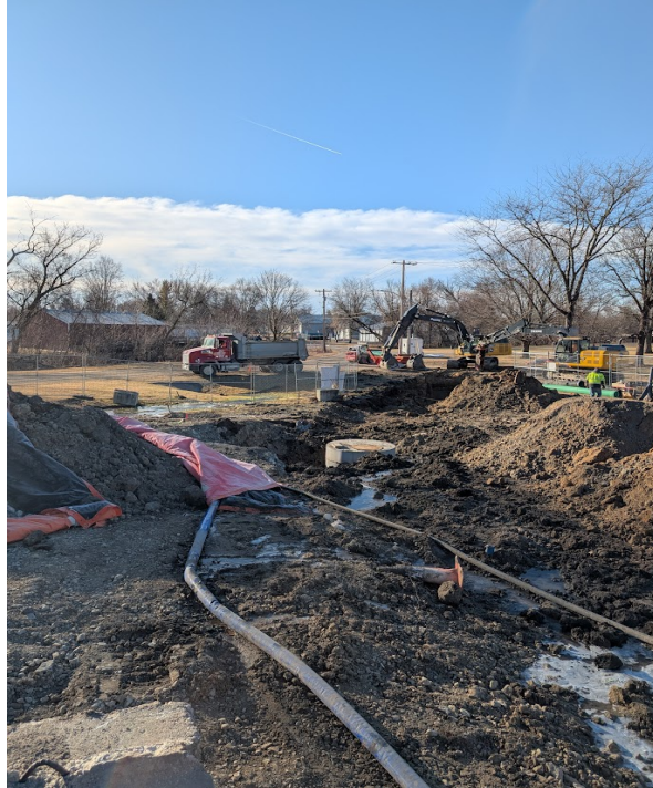
Site - excavation for gravity sewer to MH M off Hendricks St.
