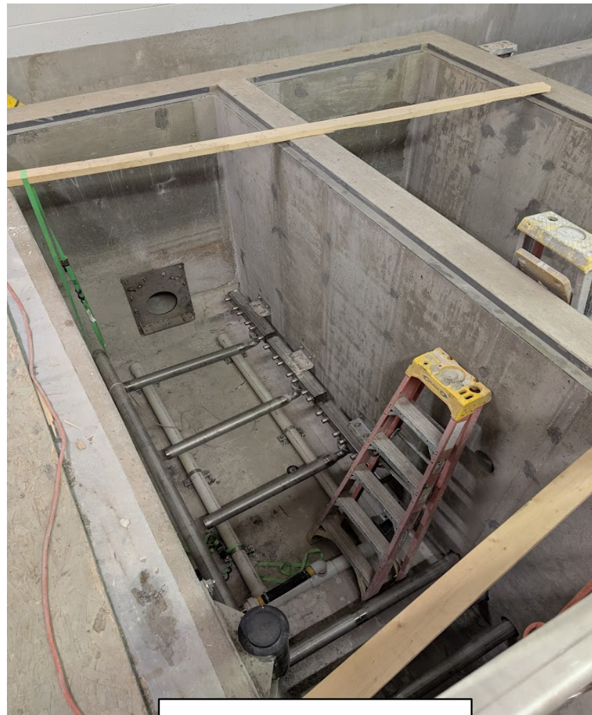
Str. 50 - New concrete walls for Tertiary Filter basins
