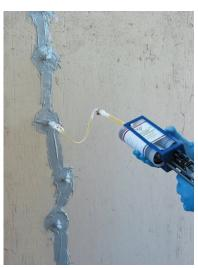
Area 4 **Crack Repair Additional Crack / Crack Injection With Other** Work **Pipe Penetration Injection**
