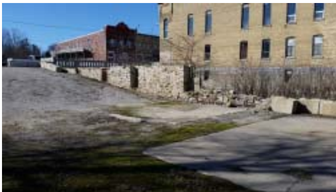
From SE cor of site looking NW
