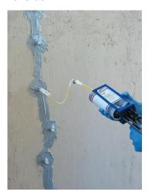
Area 4 **Crack Repair Additional Crack / Crack Injection With Other** Work **Additional Crack / Crack Injection With Other** Work
