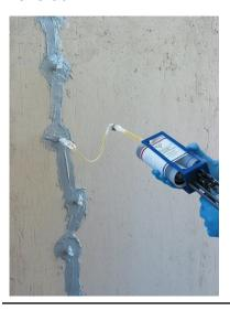
Area 3 **Crack Repair Carbon Fiber Crack Stabilization System**
