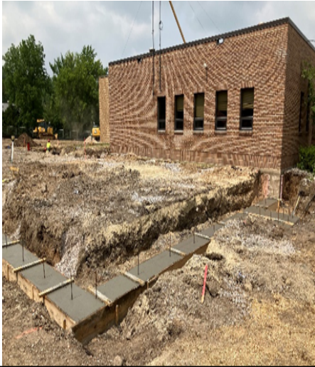
Str. 10 Concrete Footings
